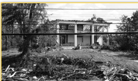
APRIL 27 Storm Damage
